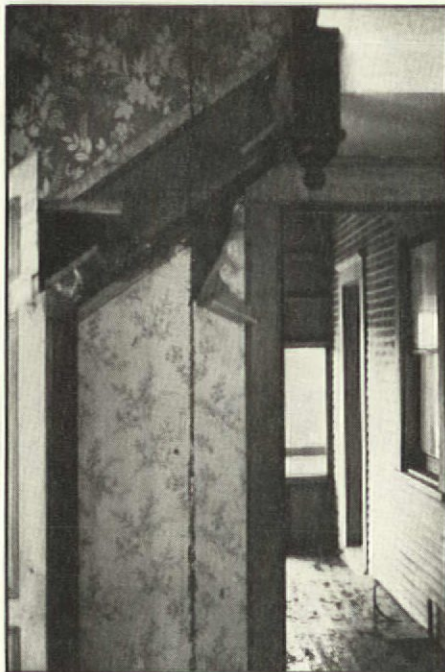
Left: No, this isn't a damaged photograph. The line you see is part of the great bifurcation performed by housemover Earl Bradford. The section of stairway was removed before the house was cut. Above: Here's half the house moving down the street. Notice the timbers propped up to support the house.
