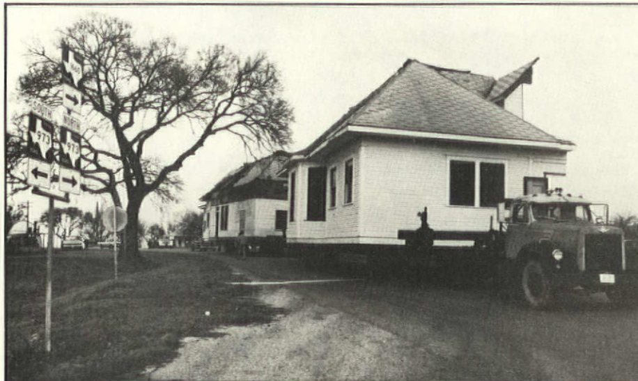
The house prepares to make a turn on its 12-mile journey to its new site.
