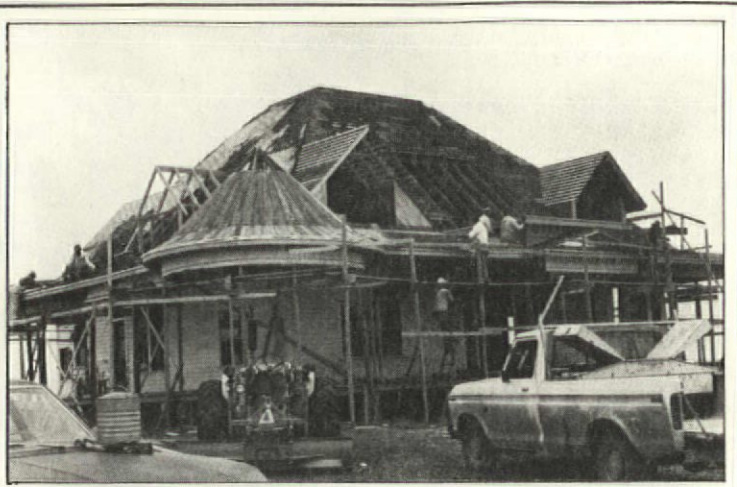
Left: The house — seen from the back — gets ready to pull itself together. Above: Once it was back in one piece, the real work on the house began. Here you see the reassembling of the verandah and the reconstruction of the dormers and balcony. Below: Does this house look familiar when seen from a distance? Picture a young woman in an old jalopy. She gets up, takes off her hat, and calls out to the man on the porch, "Travis, you're a year too late." (Incidentally, nobody who made the commercial knows what that line means either.)
