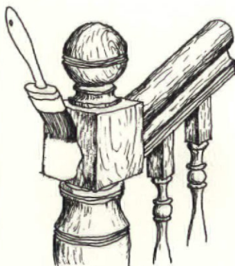
1. Apply paint thinner or special restoring solvent (see article for formula). Allow solvent to soak in for 3 minutes.
