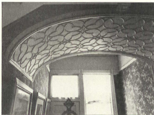
An eye-catching Anaglypta pattern on the entrance hall ceiling of the Kearney Mansion in Fresno, California.
