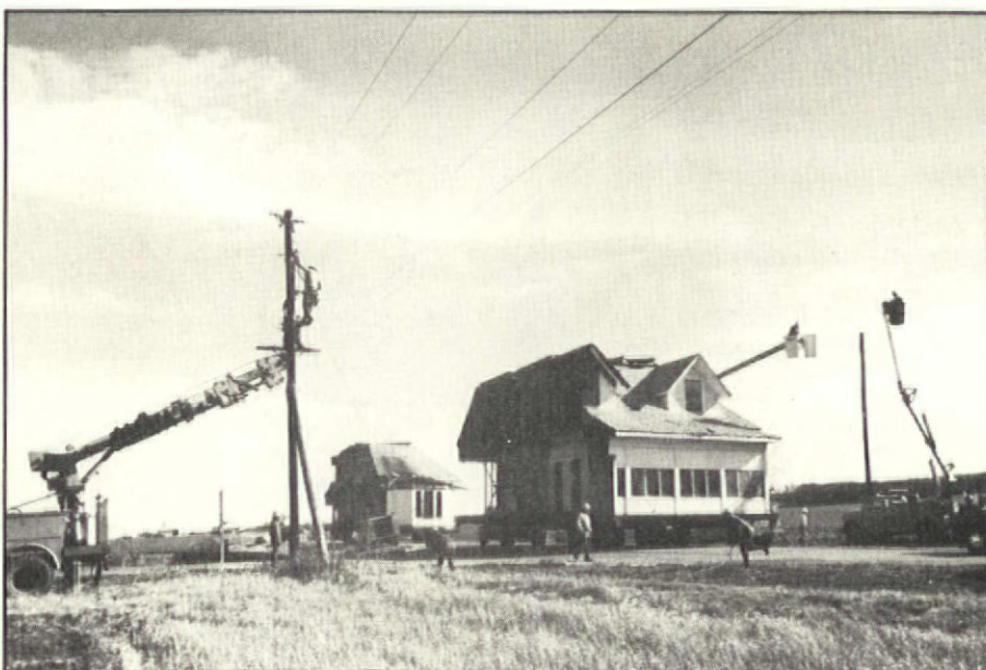
Three cherry-pickers work in the air at one time to get the house through this intersection.
