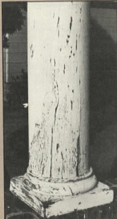
paired. Right: Water from a leak in the roof entered this column through the unflushed capital. That's all that was needed for rot to cause this extensive damage.
