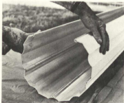
Assembling a Moultrie Column.
