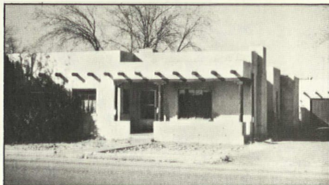
With this Pueblo house in Las Cruces, New Mexico, you can clearly see the exposed beam ends and square windows typical of the style. (Note the matching garage at right.)
