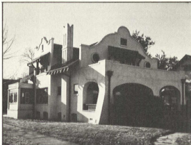
This house is a full-blown and unmistakable example of the Mission substyle, with its full mission church facade, verandah in the shape of an atrium, scalloped chimneys, and side gables. It would be nice to report that such a splendid specimen was found on its native sod (or scrub, better) somewhere in central or southern California. Alas for logical expectations -- this one was built on the Windsor side of the Detroit River, a block or two from the Ambassador Bridge! But it does show how far the magic of Hollywood glamour could carry a style.
