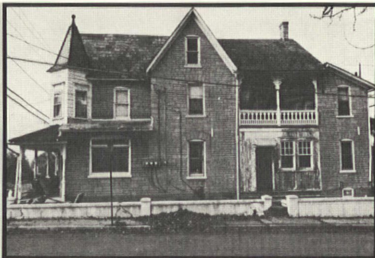
Before solar, the house was by no means untouched — that's "stonecoating." But it did have its original window openings, massing, and slate roof. And when it looked like this, of course, nobody was displaying it as the path to the future.
