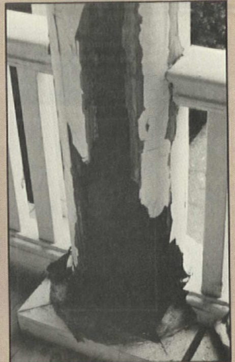
paired. Right: Water from a leak in the roof entered this column through the unflushed capital. That's all that was needed for rot to cause this extensive damage.
