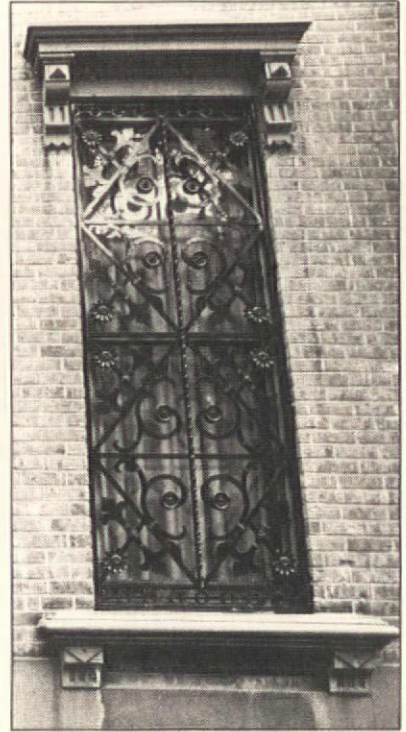
Close-up of the new window grille
