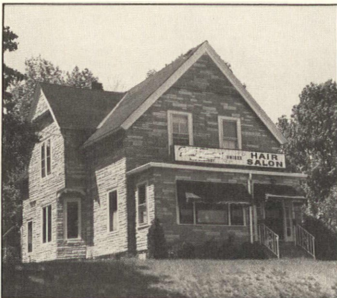
The Guidelines do not encourage covering a wooden house with fake stone in an attempt to make it look like a castle.
