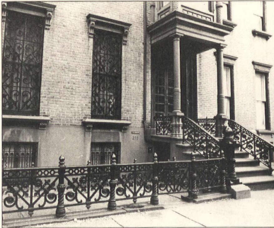
If you're in a neighborhood where window grilles are a necessity, you might consider budgeting more than usual for a set of custom-made bars. In this example, the iron-worker fabricated the bars to match the detailing of the original fence and balustrade.
