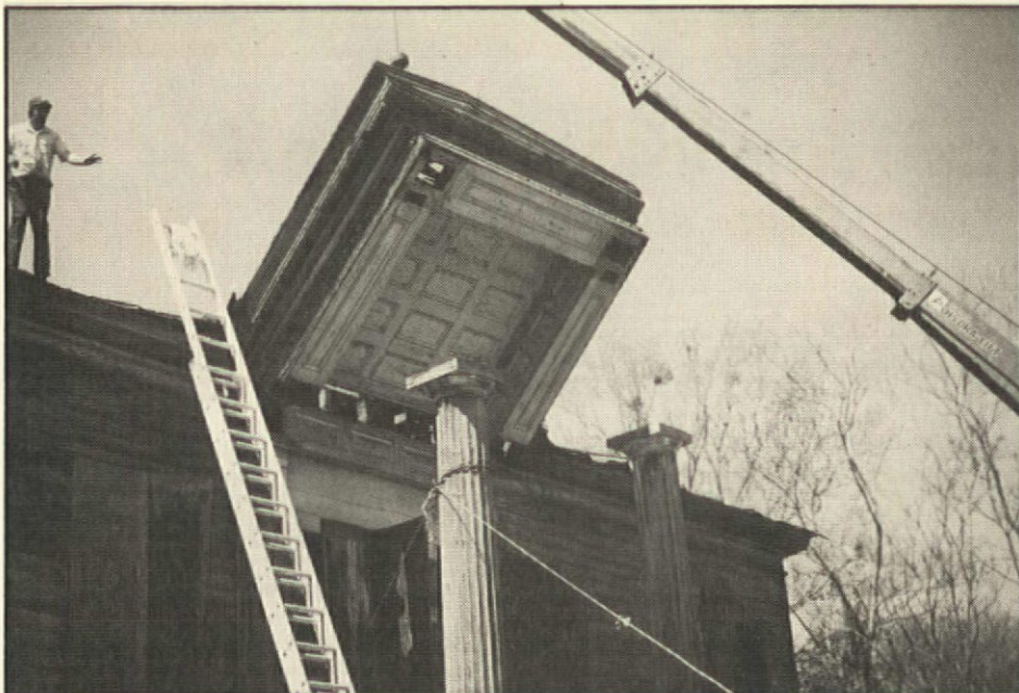
Renting a crane proved to be a simple, quick, and inexpensive way of removing both porticoes.
