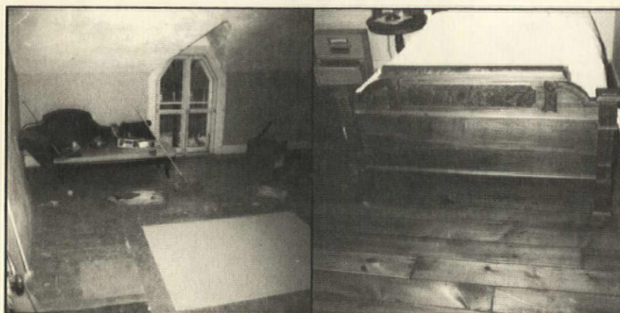
Left: The bedroom with tiles glued to the floor. Center: The same pine floor after the tiles were pried up and the
