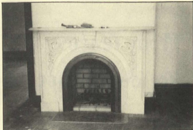
The back parlor fireplace just after reconstruction and replacement of marble mantle. The floors haven't been sanded nor the walls papered.
