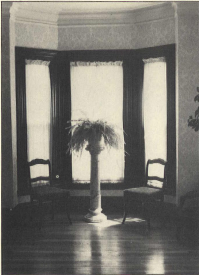
The center window of the front parlor bay had been replaced in the past with ill-fitting and incompatible materials. The Kullmans reconstructed the original. In order not to hide the woodwork, shirred curtains have been set into the windows.
