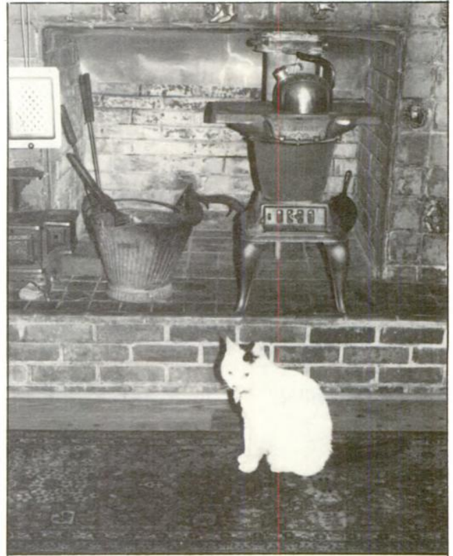
In this close-up photo of the fireplace and stove, you can see the piece of aluminum wedged in place behind the stove to direct warm air into the room.
