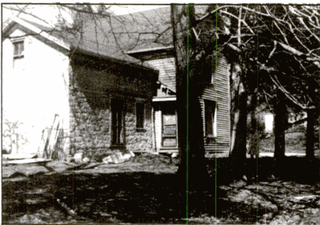
Norma's farmhouse before work began. The stone part was built in 1865 and the frame portion added about 1900.
