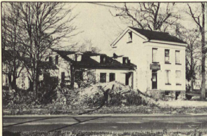
The house as it was on its original site. There had been no indication that the back wing was an addition until it began to move away from the house when it was lifted onto the wheels.
