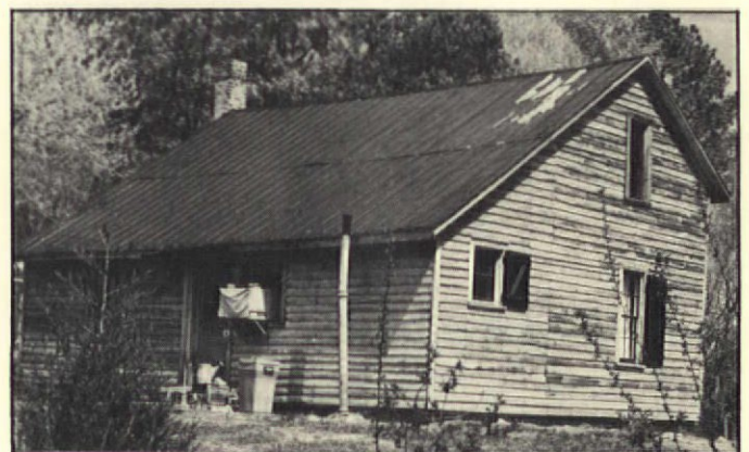
The sloping roof of the house is called "catslide"--a southern term for saltbox.
