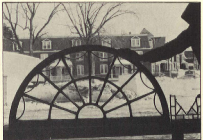
A typical Georgian style fanlight from above a front door. When glass was a scarce commodity, segmental windows such as this made very efficient use of crown glass, which was clear enough to see through although frequently wavy.
