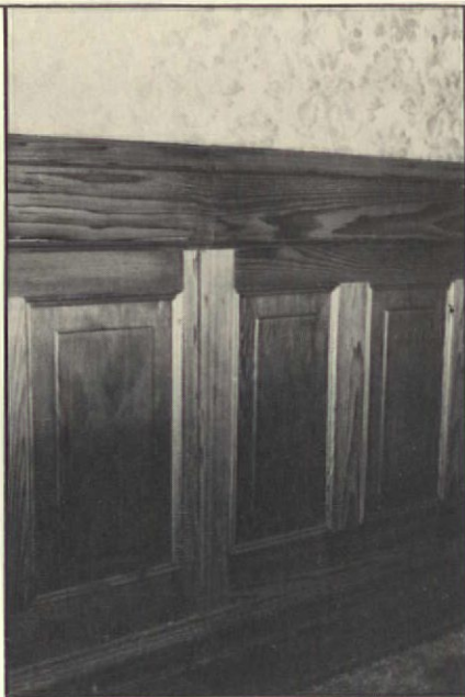
Grain in top boards did not match because of previous patching. Painted grain lines hid the mis-matching.
