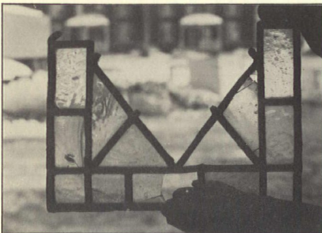
A 19th century reproduction of a medieval-type window. Note the typically geometrically shaped pieces of thick, irregular glass. Windows such as these were designed to set in casements and let in light; looking through them was rather impossible.
