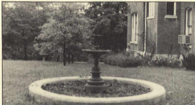
This fine example of a residential fountain is located in Anna, Illinois, and through repairs could run once more. It shows the typical cement basin that some of the iron fountains were constructed with.
