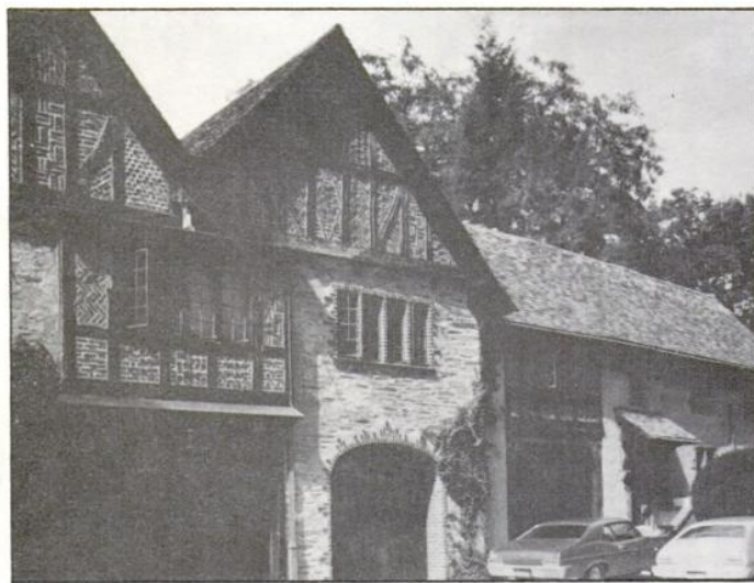
Not as commonly found in the American versions, this 1929 Pennsylvania Tudor has varying brick patterns in the "nogging" between the beams. These decorative brick patterns were often used in old English half-timbered houses.
