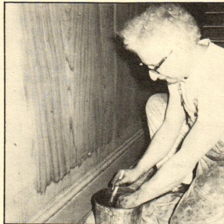
After stain has set up, graining figures are made with cotton and stain.
