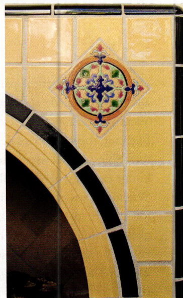
BELOW: Square deco tiles surround the firebox in a fireplace fully covered in handmade 3x6 subway tiles, all from Weaver Tile.
