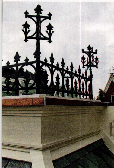
Victorian roof cresting is still made in many designs. This is a painted steel assembly from Capital Crestings: capitalcrestings.com
