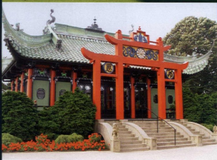
TOP: The Chinese Tea House was built for Alva Vanderbilt behind Marble House, her mansion in Newport, Rhode Island. ABOVE: Reminiscent of a southern Chinese temple, the Chinese Tea House was designed by Richard Morris Hunt's sons, both architects like their famous father. It features lacquered red gates and columns and a sweeping roofline of bright-green clay tiles.
