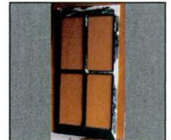
Antique window sash consolidated with LiquidWood and rebuilt with WoodEpoxy .
