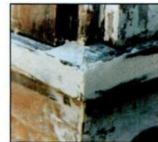
Consolidation and rebuilding of rotted windowsill with LiquidWood and WoodEpoxy .
