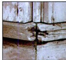
Consolidation and rebuilding of rotted windowsill with LiquidWood and WoodEpoxy .
