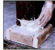
Rotted loadbearing column base sawed off and replaced with WoodEpoxy .
