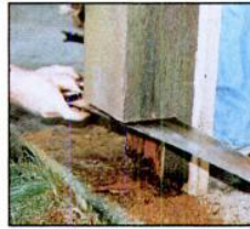
Rotted loadbearing column base sawed off and replaced with WoodEpoxy .
