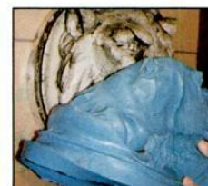
MasterMold makes molds of architectural elements in situ.
