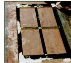
Antique window sash consolidated with LiquidWood and rebuilt with WoodEpoxy .
