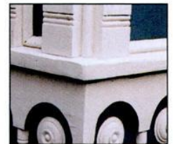
Consolidation and rebuilding of rotted windowsill with LiquidWood and WoodEpoxy .
