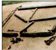
Antique window sash consolidated with LiquidWood and rebuilt with WoodEpoxy .
