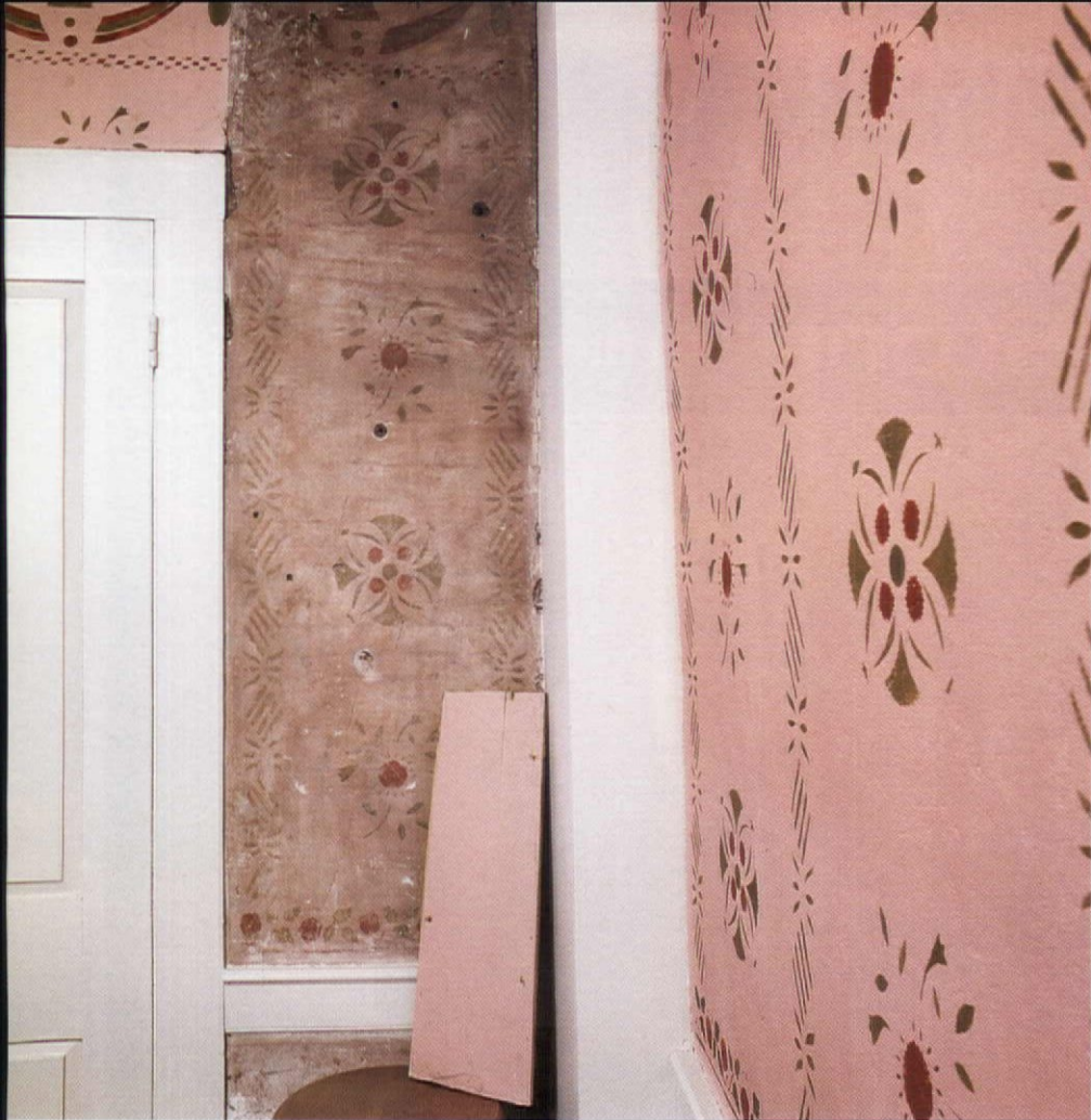
In the house's southwest parlor, you can see the re-created stenciling compared to the original panel that had been preserved. (It remains as a historic document.) The board propped in the corner was found in the house; it accurately shows the authentic salmon-color ground, to which the new color was matched.
