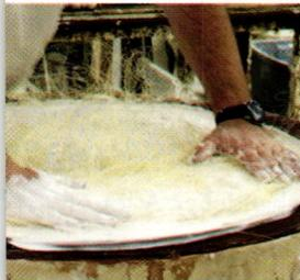
**STEP 3:** A layer of fine sisal fiber provides reinforcement. Fiber threads are stronger than woven fabric. Early plasterers knew this when they incorporated animal hair into plaster.
