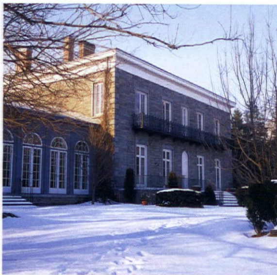
OPPOSITE: The south parlor's early-19th-century furnishings include a pianoforte by well-known maker William Geib, and a French, ormolu-decorated tripod table and chairs. LEFT: The garden façade shows a central block with flanking wings, a neoclassical design recalling the work of 16th-century architect Andrea Palladio. Renovators in 1915-18 added the fanlight transoms.
