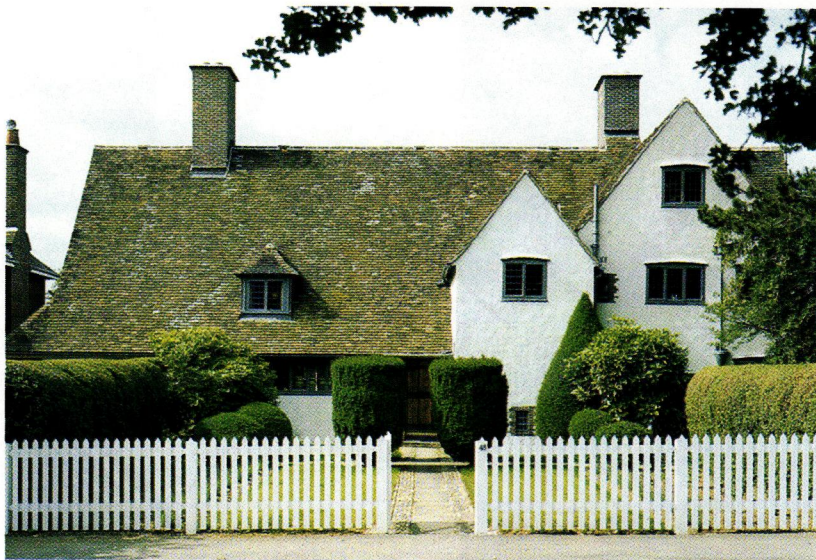
Front elevation of the house shown on page 86 by Baillie Scott, where neat formality suits the scale of this more modest suburban house.
