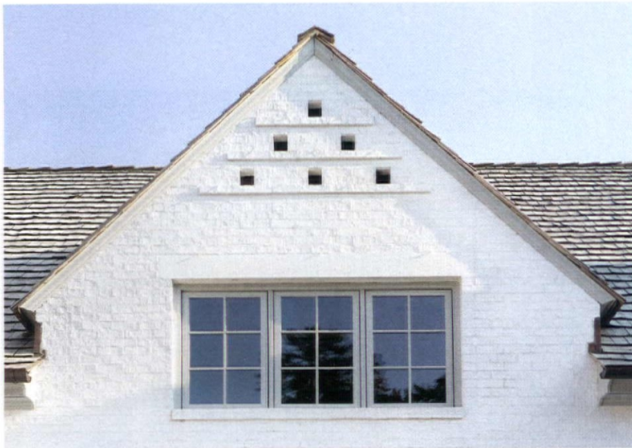
Left, top: Architect James Collins chose a brick façade with wood shingles and casement windows. Below a new old house in Texas is clad in stone.
