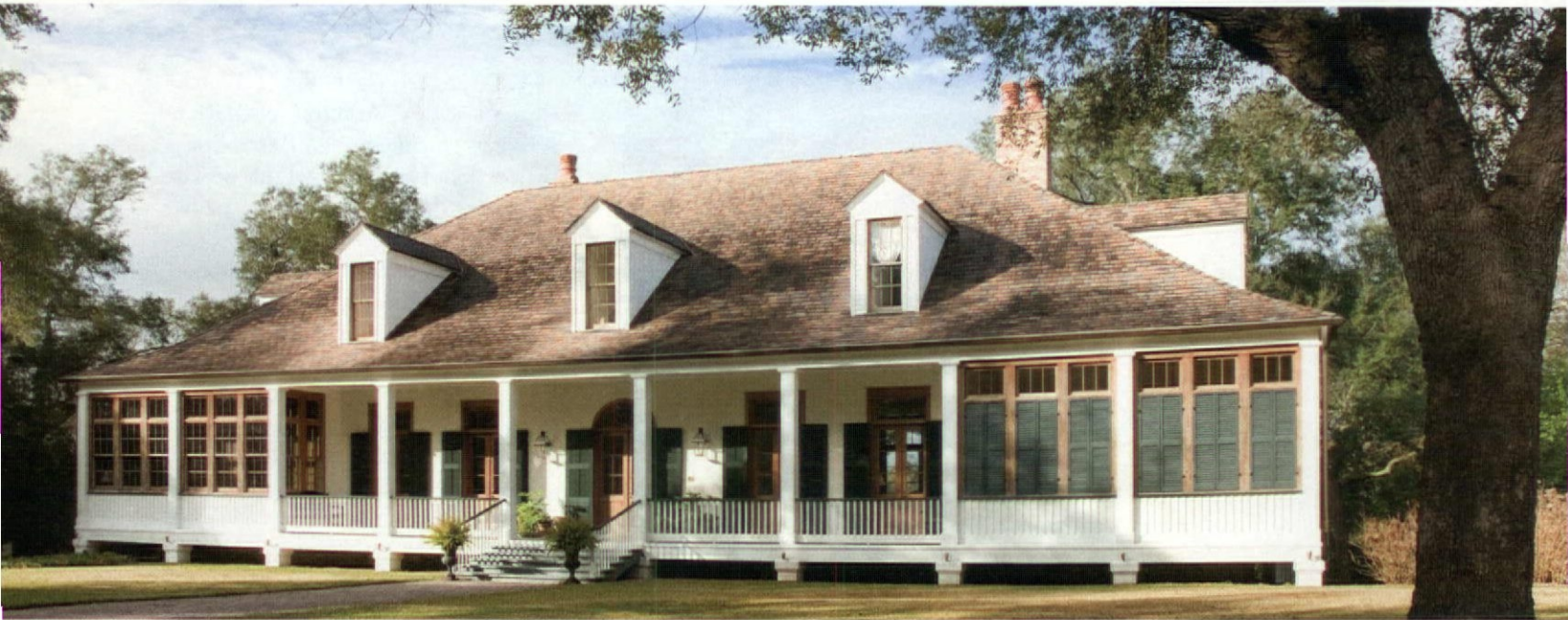
Exterior shutters keep this coastal house protected from both heat and storms.
