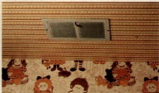
Access panel , shown in hallway at left, and register, in child's bedroom above, are only evidence of the furnace. Access panel allows for easy servicing; when panel is removed, innards of Dynaceil can be lifted out.
