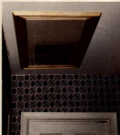
Access panel , shown in hallway at left, and register, in child's bedroom above, are only evidence of the furnace. Access panel allows for easy servicing; when panel is removed, innards of Dynaceil can be lifted out.
