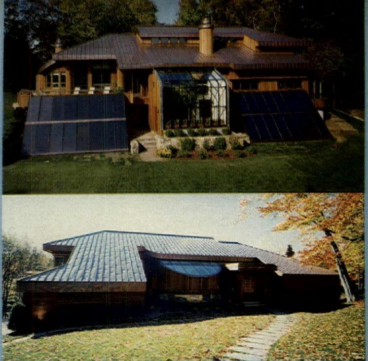
Rear elevation of Sun/Tronic house (top photo) faces south and contains two active solar collectors and a two-story passive solar greenhouse whose floor stores heat. Just inside greenhouse are the copper-tube solar collectors.
