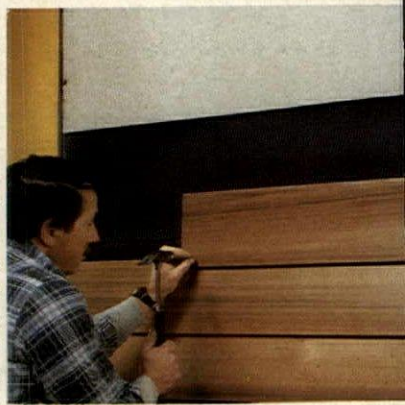
Sidewall panels provide an exterior-grade nailable surface that can be painted, as shown above, or finished with siding, as shown at right. In the latter case, a layer of building paper should be installed over the Thermasote® before the application of shingles or shakes. Other sidings can be used as recommended.
