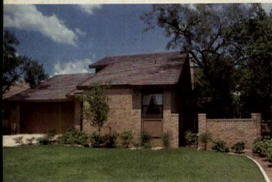
Zero-lot-line model (above) features the same concrete-tile roofing and brick exterior as the conventionally sited detached homes (previous page). Elevations vary, but all have a contemporary look. When built out, development will include a 52-unit zero-lot-line project, 72 standardized single-family homes and a few $170,000-to-$200,000 custom homes on prime lots with views of a wooded ravine.
