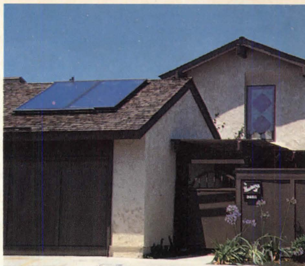
Nova™ collectors , shown installed above, are part of a hot water system that can heat jacuzzis and pools. American Home Solar Systems. Circle 211 on reader service card
