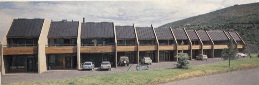
Energy-efficient townhouses feature concentration of glass on south elevation ( see left ). Units also come equipped with woodburning stoves, R-19 insulation in walls and R-30 in ceilings. Although living area in one-bedroom unit ( photo below ) measures only 576 sq. ft., volume ceiling and open loft area help create spacious feeling.
