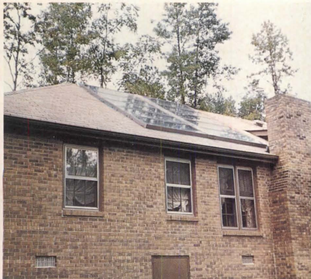
Flatplate collectors , shown installed above, are constructed of double-glazed tempered glass, inch-thick insulation, copper tube and plate, and an aluminum frame. National Solar Supply. Circle 216 on reader service card
