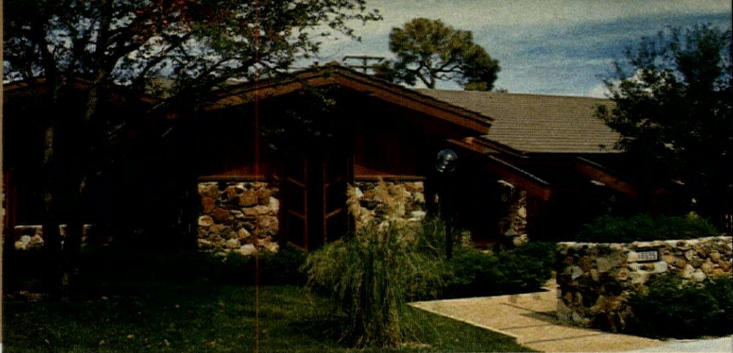
Original house (above) had already had garage converted to living area when photo was taken. New stone-and-wood facing (right) replaces original CBS facade.
