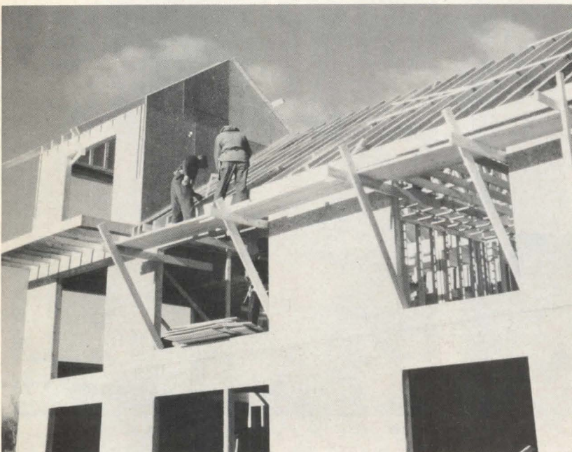
"Norbord" wafers (above) consists of wood flakes bonded together with wax and a waterproof resin. Product is presently available in eastern and central Canada and northeastern U.S. Northwood. Circle 240 on reader service card
