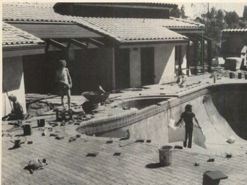
Concrete paving stones (above) are interlocking modules that can be installed over a concrete or aggregate base. Grouting is not required. Four patterns are available in earthtone colors. Low-maintenance stones absorb less than 5% of moisture. Muller Supply. Circle 232 on reader service card
