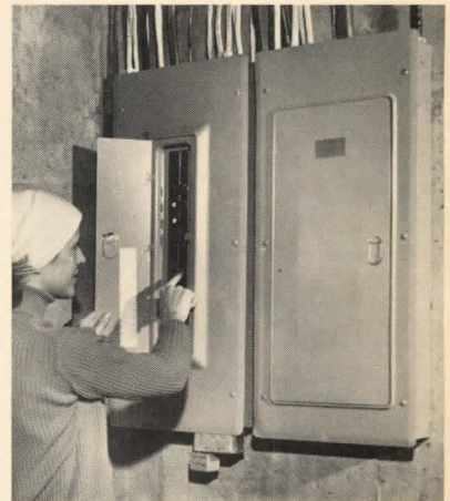
Two 200-amp load centers (above) are used as an alternate to a single 400-amp center, eliminating need for 3" conduit. Load centers have push-button circuit breakers that have thermal and magnetic protection against short circuits and overloads. Gould. Circle 233 on reader service card
