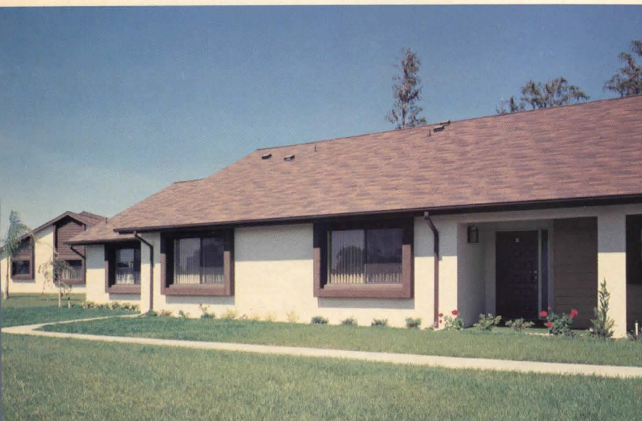
Village on the Green, Clearwater, Florida. Frank Macagnone, Division President, U.S. Home Corporation
