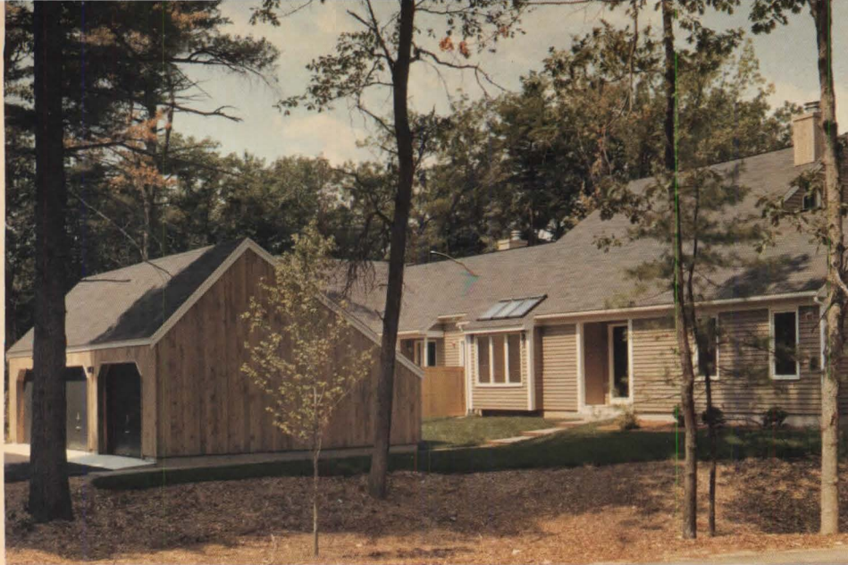
Entry courts of attached houses are screened by detached garages and wooden privacy fences.
