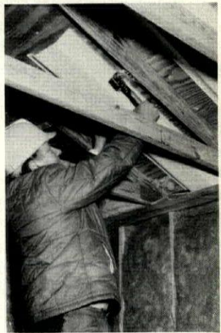
Metal lath (left) is backed with a polyethylene film so that lath and film barrier go up simultaneously. The lath can act as a base for machine-applied plaster in non-load-bearing walls. USG, Chicago. Circle 236 on reader service card
