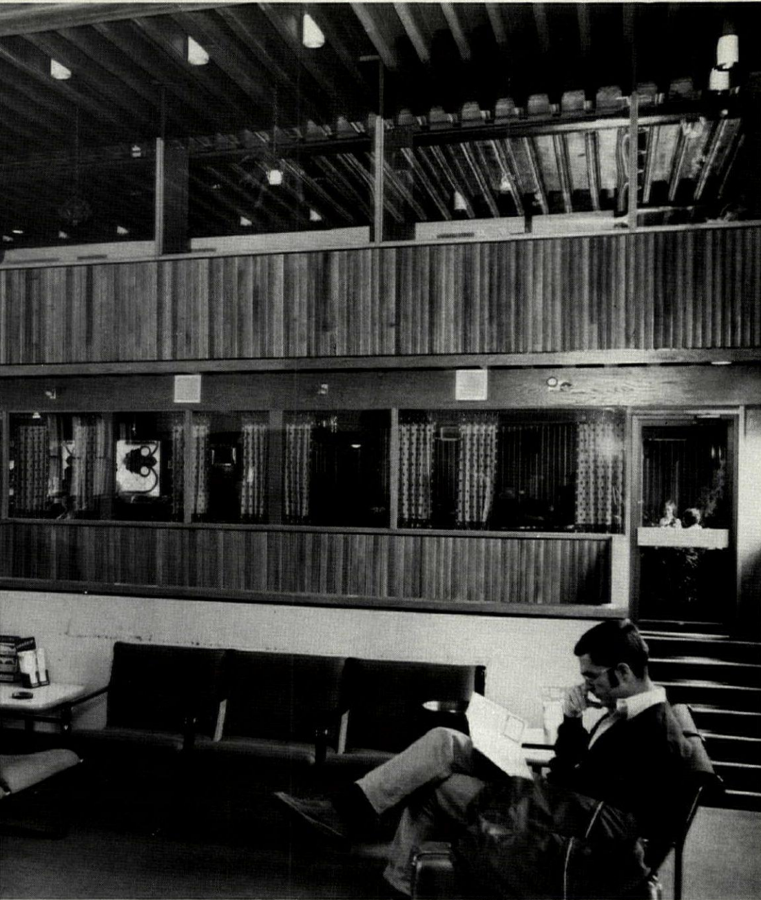
Waiting room (photo left) was cut in half to make room for a restaurant (background) and a second waiting room was provided at basement level. This is reached via a new staircase (see "before" picture facing page and "after" picture below left). This staircase also leads to the train platform (not shown), which is a half level below the main waiting room. A mezzanine level was added to provide additional restaurant and office space (section below). Both staircase and mezzanine were paneled with wainscoting salvaged from the building.
