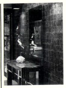
Ceramic tile, Renaissance<sup>TM</sup> (above), is suitable for application on interior walls and countertops. Available in 41/4"x41/4" and 6"x6" sizes, glazed tiles come in copper, bronze, gold and olive. Easy-to-clean, 5/16" thick tiles can be used with colorcoordinated grout. American Olean Tile, Lansdale, PA. Circle 218 on reader service card
