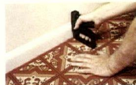
Tredway installs with staples.
