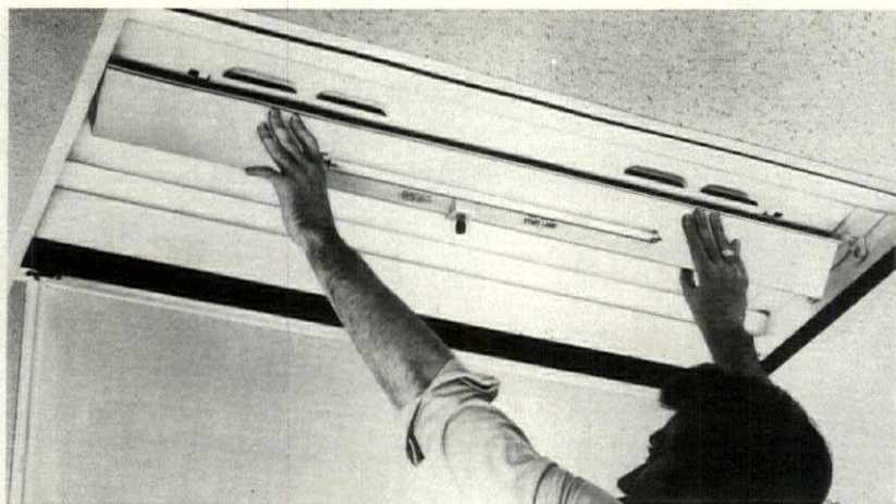
Emergency lighting assembly (above) fits into a standard fluorescent troffer. In case of a power failure, a battery-powered lamp that provides illumination for up to 90 minutes automatically switches on. Keene, Wilmington, MA. Circle 230 on reader service card
