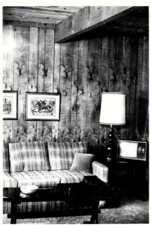
Aspen plywood paneling (above) is prestained in one of six weather-look finishes. Paneling, which is 1/4" thick, can be applied easily with nails or adhesive and is moisture and heat resistant. Iron Wood Products, Bessemer, MI. Circle 221 on reader service card
