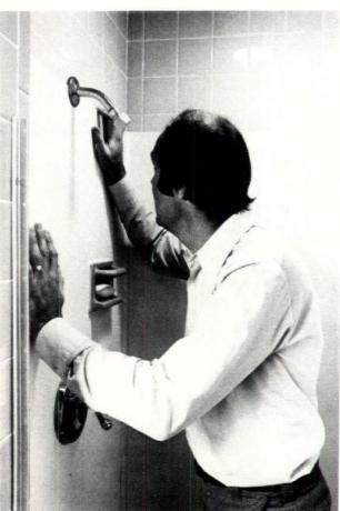
"Shower Shield" (above), waterproof sheet material for shower stalls, tub surrounds and bathroom walls, installs quickly without special tools. Lightweight, 1/25"-thick wallcovering has white stain-resistant finish. Consolidated, Canal Fulton, OH. Circle 204 on reader service card
