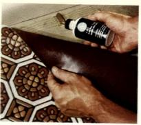
Tredway installs over concrete with a band of adhesive.
