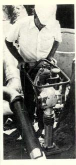
Portable rammer/compactor (above) is easy to maneuver in narrow trenches. A 6" shoe is standard. A narrow 4" shoe with a 12" extension is optional. Wacker, Milwaukee, Wis. Circle 345 on reader service card
