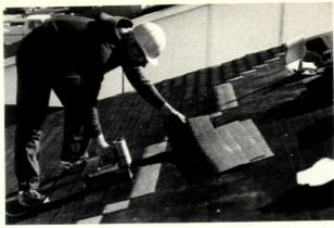
Roofing stapler (above) is designed for shingle applications. Unit has "E-Z Clear" feature that eliminates downtime caused by fastener jams. Senco, Cincinnati. NAHB booth 1024. Circle 356 on reader service card
