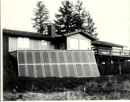
Modular solar collectors (above) are prepackaged, prepiped units suitable for use on new or existing construction. The collector plate is constructed of copper sheet for highest heat transfer efficiency and best corrosion resistance. Unit has transparent cover, insulated housing and simple piping connections. Revere, New York City. Circle 343 on reader service
