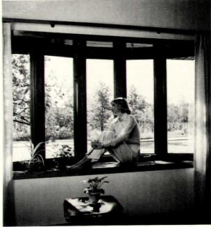
Casement bow window (above) features concealed hinges. Complete with seat and head boards, windows are equipped with smooth "Rotogear" operators and double sash locks. Unit features double weatherstripping. Marvin, Warroad, Minn. NAHB booth 2728. Circle 299 on reader service card
