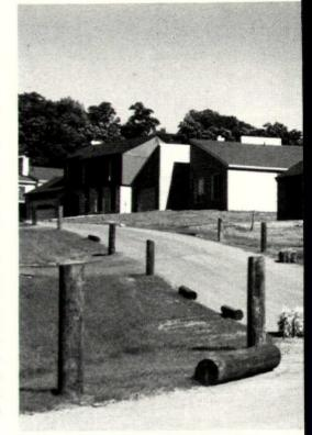
Bollards substituted for curbs in photo above keep traffic from running up on property and mark pavement limits for snowplowing.
