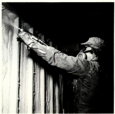
Portable sprayer system (above) is designed for applying plural component materials such as silicone and urethane. A solid state electronic system allows choice of application methods plus control of pressure and temperature. Galvo, Kohler, Wis. CIRCLE 242 ON READER SERVICE CARD
