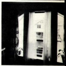
Aluminum-framed thermal windows (above), used throughout complex, conserve energy and reduce interior condensation. Windows' heat- and cold-retention is estimated to save about \$9,000 a year over new, single-glazed aluminum windows at current fuel
