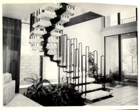
Staircase center beam (above) is constructed of 31-lb steel elements secured by locking device. No clamps or screws are visible. Elements can be used for curved or straight configurations. A T Univ-Stairs, Chatsworth, Calif. CIRCLE 202 ON READER SERVICE CARD
