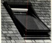
Roof window (above) affords more daylight than vertical dormers of same size. Constructed of pine, window rotates 180°. Weatherproof window has insulated glass. Velux America, Woburn, Mass. CIRCLE 219 ON READER SERVICE CARD
