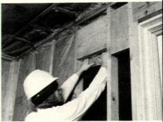
When using faced insulation in an are where there is blocking, push a section the insulation behind the blocking an staple the insulation to the top plate and t the bottom of the nailer. Then insulate th balance of the space by butting another ba to the piece behind the blocking.
