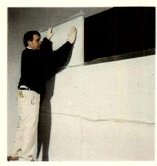
A plasterer demonstrates the ease and simplicity of the Thermoclad system, applied here over an 8 x 8 foot panel of exterior gypsum over metal studding. In the first photo, Thermoclad insulation
