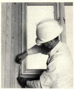
Cracks around windows and doors are a major source of air infiltration. These voids should be chinked with liberal amounts of insulation. If cracks are too small to permit chinking, fill them with heavy caulking.
