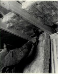
hen using a double layer of batts to insue the attic (above), push the top batt beeen the chords first. Use the bottom batt push the top one into place and staple it the ends and sides. Make sure the top tts are level and butt tightly. (Note: to inease insulation efficiency in the attic area, ild a plywood frame around the scuttle le and place insulation—the same ickness as used in the attic-over the uttle-hole cover board.)
