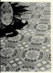
Natural stone tiles, "Alta Quartzite," are used to dress up a patio. The material, which absorbs almost no water, is immune to cracking due to freezing and thawing. Grey-green tiles are resistant to mildew. Gran-Quartz, Tucker, Ga. CIRCLE 239 ON READER SERVICE CARD
