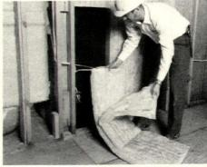
In stud spaces containing wiring or outle boxes, split the insulation, forcing half b hind the wires and box. Then install the front half of the insulation in the conver tional manner, making sure the piece re moved to accommodate the box is cut for tight fit.
