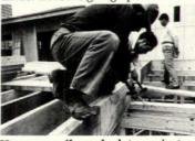
**Hammer-nail method** is replacing Japan's system of mortised joints.
