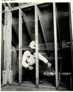
In attic knee walls, staple three bands of 8 wide polyethylene to the back of the stud to help prevent insulation from being pushed back too far.
