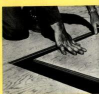
The panels have a preciselyneered tongue and groove joint
