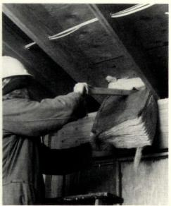
After the cardboard sleeve is in place, force in the insulation, with vapor barrier face up. Make sure the insulation fully covers the top plate.
