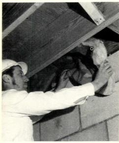
Here, perimeter insulation is installed parallel to the joists. After stapling the batt end to the sill along the band joist, wedge the insulation lengthwise between the plate and the subflooring.
