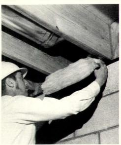
To insulate between ends of the joists, cut a length of batt to fit in the configuration in the spaces. Then staple it to the subflooring and at the sides of the joist.
