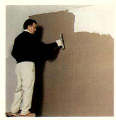
with its factory laminated fiberglass mesh, is applied to the gypsum board. In the second photo, the strong, cementitious prime coat is troweled over the insulation. And in the third photo, the
