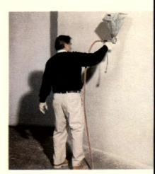
attractive, textured finish coat is sprayed over the prime coat. Both prime and finish coats can be troweled or sprayed. The result is superior insulation and the attractive finish shown at the right.
