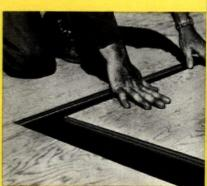
The panels have a preciselyneered tongue and groove joint eliminates the need for king. Another big time-saver. And the surface is so smooth resilient tile, linoleum, eting and hardwood flooring can laced right over the plywood. 2.4.1 Single Floor. One of the t plywood moments.
