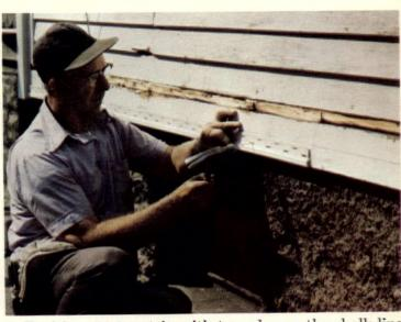
Position starter strip with top edge on the chalk line. Do not nail too tight; stop when hammer head touches edges of nailing strips.
