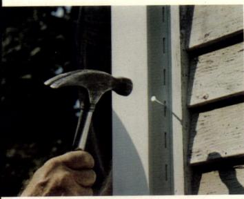
Install all inside and outside corner posts. Leave 1/4" top. Finish nailing every 10" to 12" in the center
