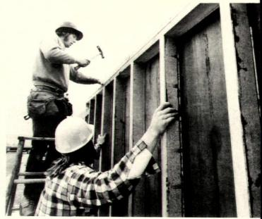
**Composite 2x4**, "COM-PLY," consists of a core of  $1\frac{1}{2}$ "x2 $\frac{5}{6}$ " strips of particle board with  $\frac{1}{16}$ " high-strength solid wood veneer laminated to each narrow side. Straight, durable studs are easy to nail. Georgia-Pacific, Portland, Or CIRCLE 256 ON READER SERVICE CARD
