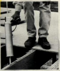
field-glued plywood single floor.
