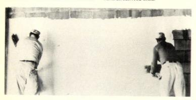
One-step system for insulating and finishing concrete or masonry walls, "InsulWal" (right), consists of a sandwich panel of urethane foam between gypsum board and foil plus a proprietary adhesive and special clip mechanical fastener (shown). Panel-Era, Salt Lake City. CIRCLE 252 ON READER SERVICE CARD
