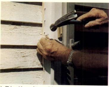
4. Trim sides and tops of doors and windows with J channels or window/door caps. Installation of siding panels now begins.
