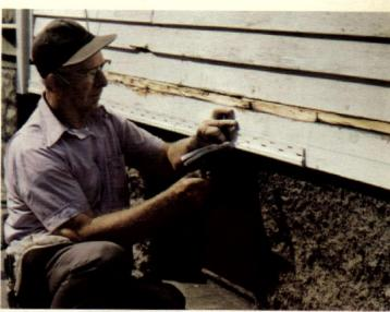
3. Position starter strip with top edge on the chalk line. Do not nail too tight; stop when hammer head touches edges of nailing strips.
