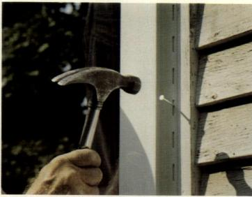
2. Install all inside and outside corner posts. Leave  $\frac{1}{4}$ " at top. Finish nailing every 10" to 12" in the center of the slots.
