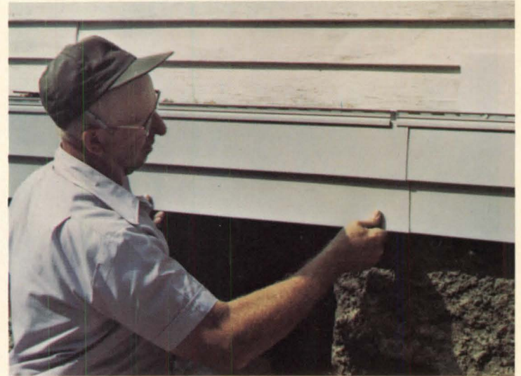
5. Snap bottom panels into the starter strip and nail. Backer board can be used for extra insulation.
