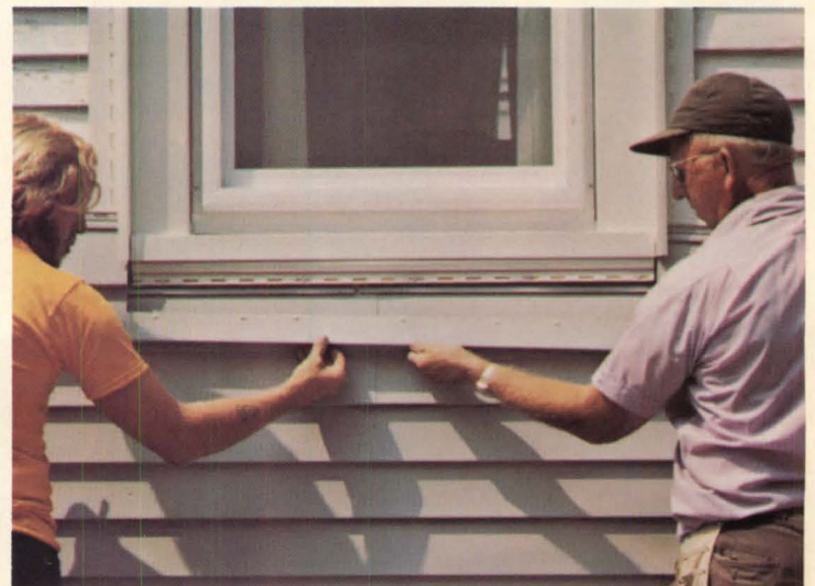
9. Slide the panel into the undersill trim. Installation of the top course follows a similar procedure.
