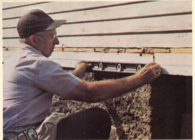
1. Check to see that all sidewalls and base are level and plumb. Snap chalk line for the starter strip.
