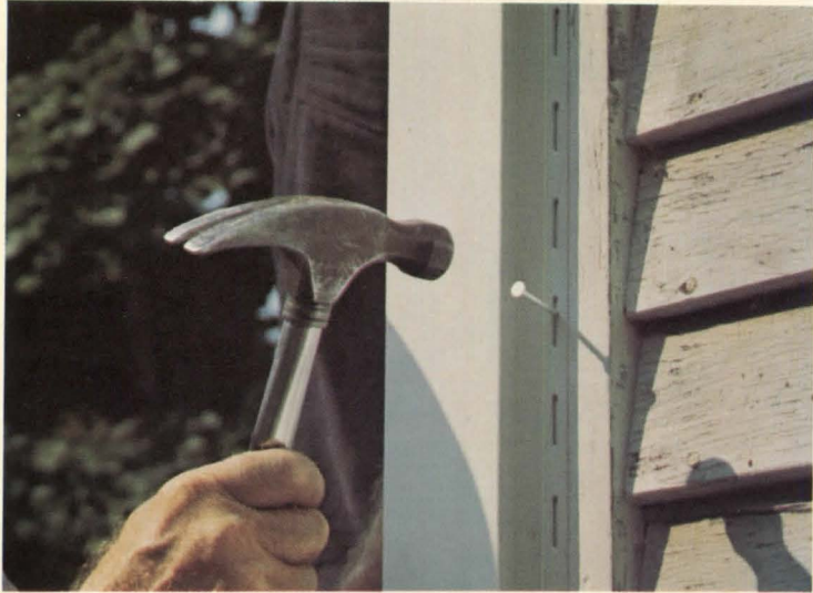
2. Install all inside and outside corner posts. Leave \frac{1}{4} " at top. Finish nailing every 10" to 12" in the center of the slots.
