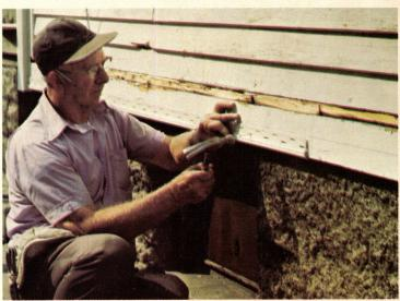
3. Position starter strip with top edge on the chalk line. Do not nail too tight; stop when hammer head touches edges of nailing strips.
