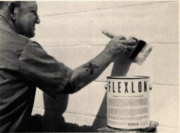
Liquid plastic coating, "Flexlon #3," is waterproof, fire retardant and flexible. Interior/exterior compound may be used on all common building materials and on exposed polyurethane-foam insulating surfaces. Coating cures dust-free in 30 minutes and expands and contracts with surface it is bonded to. Weber & Sons, Freehold, N.J. CIRCLE 259 ON READER SERVICE CARD
