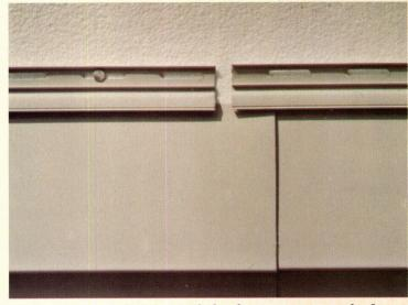
7. Overlap panels by ½ of the factory pre-notched cutouts. Leave ½ inch space between the nailing strips.
