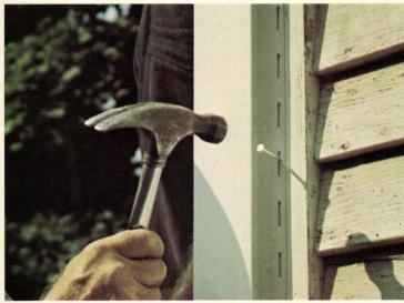
2. Install all inside and outside corner posts. Leave ¼" at top. Finish nailing every 10" to 12" in the center of the slots.
