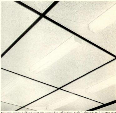
Energy-saver ceiling system provides effective task lighting at 2 watts per sq. ft. Key to the ceiling's lighting performance is the Percepta® luminaire, a twin-beam unit that eliminates reflections and reflected glares. System with a Snap-Track™ grid runner and snap-together troffers is easy to install. Holopane, Denver, Colo. CIRCLE 249 ON READER SERVICE CARD
