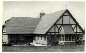
THOROSEAL PLASTER MIX applied by trowel and stipple brush achieved the old European atmosphere of the barns of the original Clydesdale breeders. The effect was accomplished by troweling on a thin, tight coat of cement-based THOROSEAL PLASTER MIX, letting it cure for a week then doubling back with another thin coat and textured with a stipple brush.
