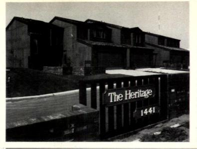
Townhouses, shown from entry sid at left and from rear, below, hav rough-sawn plywood siding ac cented with heavy wood beams shake roofs and brick chimneysradical design departure in Wichit for-sale housing. Each townhous group-either four or five unitsfeatures several plans to increas visual variety. The photo below shows how unit-to-unit privacy i achieved by walling in outdoor liv ing areas. The project's pool is see in foreground.
