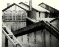
Sheath with Thermo-ply and gain valuable reflective insulation as a bonus. Thermo-ply's insulative properties can reduce the amount of mass insulation in your walls. Save in other ways, too . . . no corner bracing, less waste, fewer fasteners, easier handling. FHA accepted and code approved.
