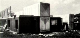
The modules contain kitchens, bathrooms, HVAC, electrical service and distribution, plumbing, fire protection and acoustical items.
