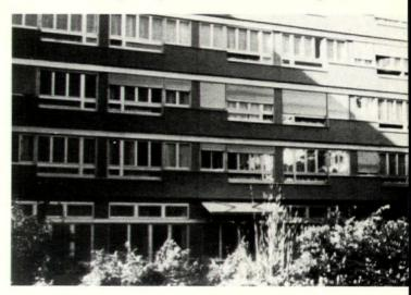
These are outside shutters that operate from inside. Made by Amrol Corporation of New Castl Indiana, they control daylight and are a deterrer to intruders. Horizontal slats made of Geon vin wind on or off a reel, which is turned by hand or ele tric motor. For more information about Geon ving in building products, ask B.F.Goodrich Chemic Company, Dept. H-33, 6100 Oak Tree Boulevar Cleveland, Ohio 44131.
