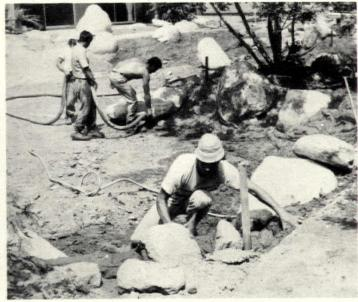
**8.** Earth-colored concrete is pumped between boulders along shoreline to hold them in place and to keep the shoreline from eroding.
