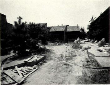
**6.** Flatwork—concrete sidewalks, steps, bridges, etc.—is installed prior to finish grading. Photo above shows walks bordering stream bed.
