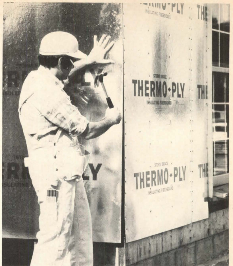
Structural insulating sheathing board, "Thermo-ply" (above), is comprised of long-fibered, specially treated plies bonded for water and weather resistance. Reflective aluminum foil is pressure laminated on both sides. Simplex Industries, Wixom, Mich.
