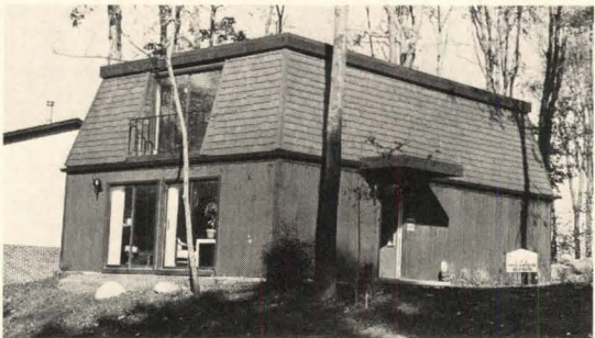
1,694-sq.-ft. two-story with four bedrooms, two baths sells for $27,900. Builder is APZ General Contractors.
