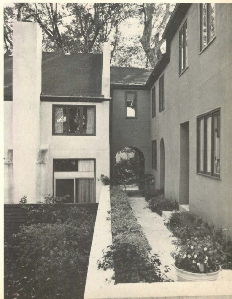
Old house ( inset photo, above ) underwent facelifting as well as structural changes during its conversion into two condo units. Roofline in converted house ( foreground, above ) was lowered and roofs of new units ( background ) built at a steep pitch to keep old and new construction in scale.
