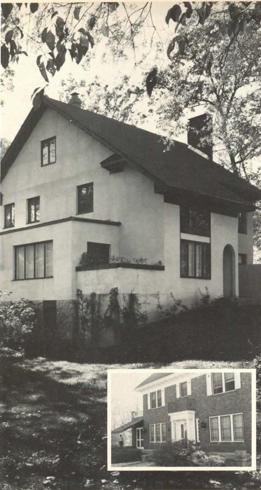
Old house ( inset photo, above ) underwent facelifting as well as structural changes during its conversion into two condo units. Roofline in converted house ( foreground, above ) was lowered and roofs of new units ( background ) built at a steep pitch to keep old and new construction in scale.
