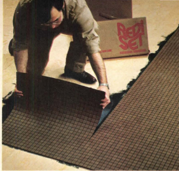
lay the pregrouted sheets,
