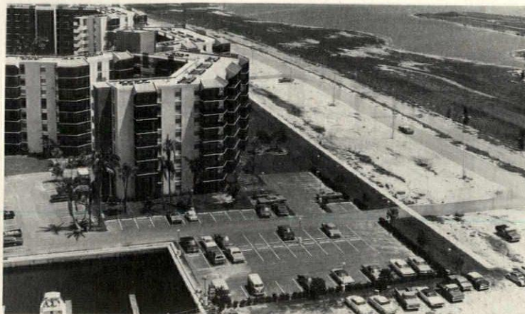
Typical condominium lease deal is offered by the Aventura development on Biscayne Bay in north Dade County, Fla. The land is conveyed with the apartments, but the recreational facilities are under lease, and the rentals are tied to cost-of-living index.
