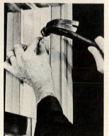
Easy-to-install window channels seal out wind, stop rattles and conserve fuel. White vinyl-finished aluminum and stainless steel channels are designed to fit standard sashes. The simple four-step installation process is shown. Quaker Mfg., Sharon Hill, Pa. CIRCLE 228 ON READER SERVICE CARD
