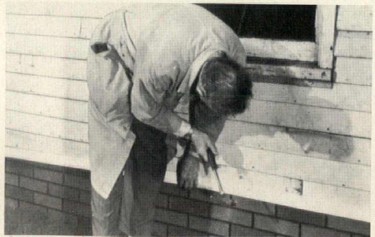
4. Starter strip. Install strip along the bottom of the building, allowing \frac{1}{4} " at the corner posts and channels. Keep ends of starter strip at least \frac{1}{4} " apart.
