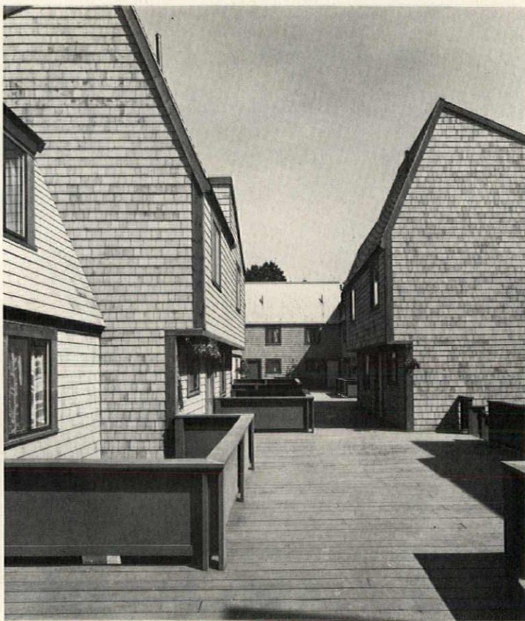
Common deck, seen here from entry end of cluster, provides access to houses. Fences enclose openings that let light into area below.
