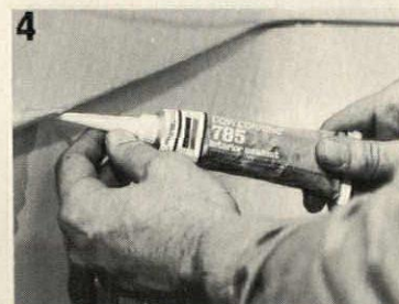
Unitized bath/shower can be installed in a standard 5' bathing alcove. Fiber glass "Versa Bath" has a Miracril acrylic surface. The four-piece system installs directly to studs. First the bathing unit is positioned and secured, then the center (1) and end (2) wall panels are mounted using special fasteners (3) that grip the stud with metal teeth. A mildew-resistant silicone-base sealant for seams provides color-matched finishing. The system, with integral safety-grip bar, soap-dish and shampoo-shelf, comes in a range of colors. Borg-Warner, Mansfield, Ohio. CIRCLE 203 ON READER SERVICE CARD
