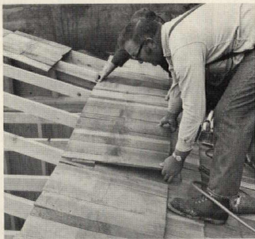
Apply both shakes and sheathing at once
