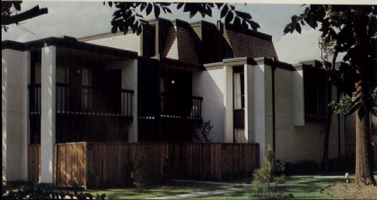
Mansard roof shows influence of French architectural style on which the Tuileries—whose name was taken from the French palace—is based. Photo above shows the swimming pool area. Fences and wing walls (left) provide maximum privacy for the project, whose density is 32 units to the acre. Architect was Kirby-Mayer & Associates Inc.
