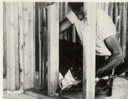
The CN-137 toenails studs to base plate ... then applies plywood roof deck.
