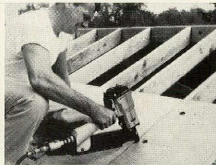
The CN-137 toenails studs to base plate ... then applies plywood roof deck.
