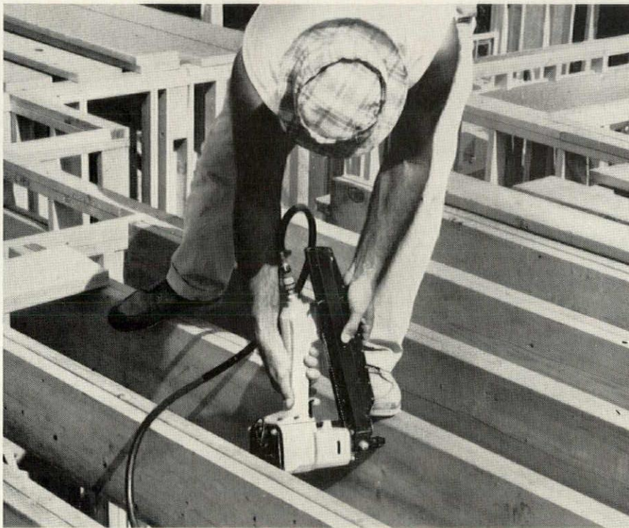
The CN-137 toenails studs to base plate ... then applies plywood roof deck.
