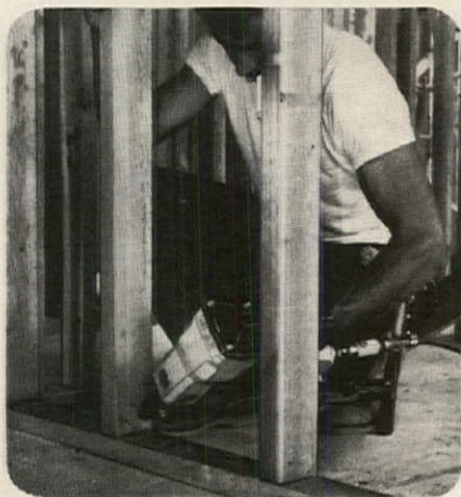
CN-137 makes fast work of toe-nailing
