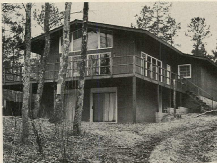
Dream house built by Ned North in Georgia's Four Seasons turned into a bad dream when he couldn't get a water tie-in. The house has stood empty since November 1970.
