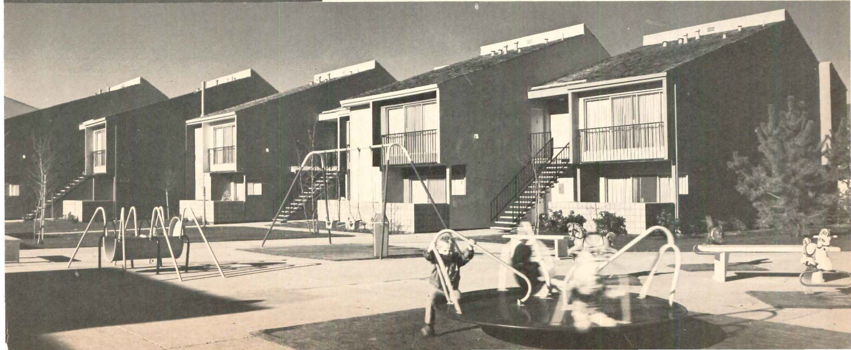
Combination plan (A and B) for three-story buildings puts a pair of two-level townhouse-type units above each one-level apartment. Other one-level apartments (C, D, E) are in two-story buildings (below), which are staggered for visual interest and privacy and are faced into courtyard for easy supervision of children at play.
