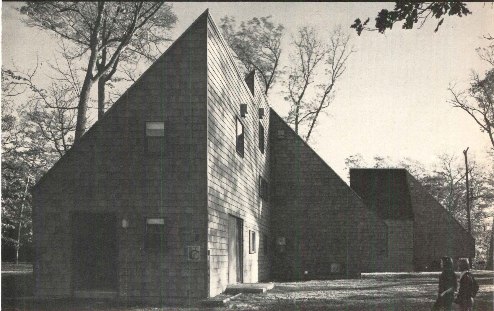
Dormitory, Bradford Junior College, Haverill, Massachusetts. Certigrade shingles No. 1 Grade, 16" Fivex. Architects: Campbell, Aldrich & Nulty. Builder: C & L Construction.
