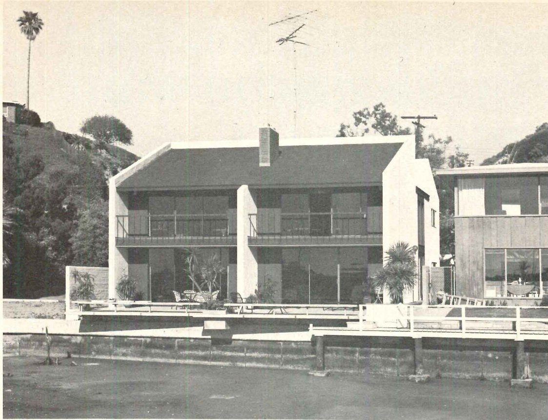
Remodeled duplex has two-story units with balconies that take advantage of the waterfront views.
